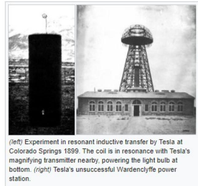
(left) Experiment in resonant inductive transfer by Tesla at Colorado Springs 1899. The coil is in resonance with Tesla's magnifying transmitter nearby, powering the light bulb at bottom. (right) Tesla's unsuccessful Wardenclyffe power station.
