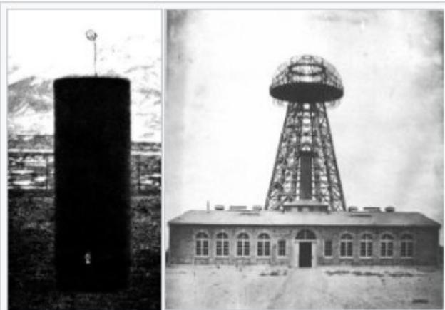
*(left)* Experiment in resonant inductive transfer by Tesla at Colorado Springs 1899. The coil is in resonance with Tesla's magnifying transmitter nearby, powering the light bulb at bottom. *(right)* Tesla's unsuccessful Wardenclyffe power station.
