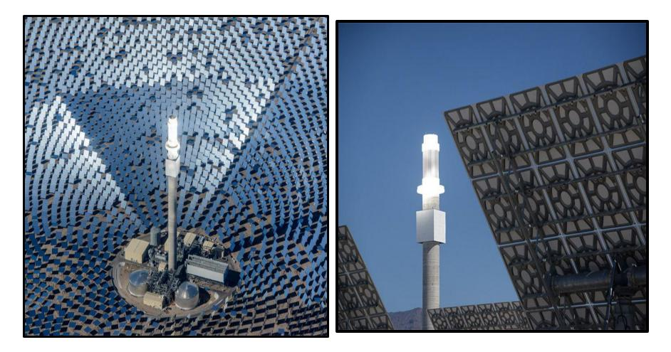
Molten salt is heated to 1000 degrees, stored, then used at nighttime to make steam to power a generator. Tower plus receiver height typically 640 feet.
